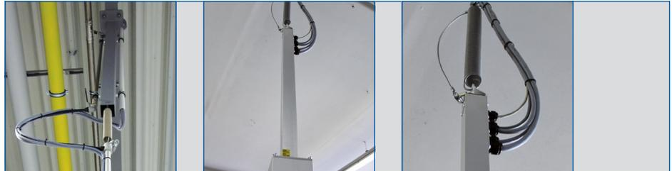
The E-BOX is attached to the ceiling or mounted to an on-site profile using a special fastening set.
