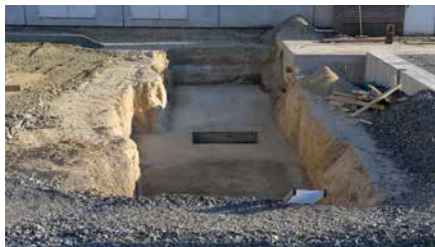
The base slab is concreted on site in accordance with specifications.
