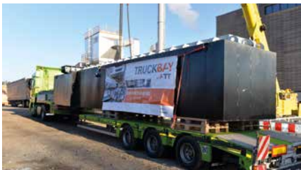
Delivery of the ready-made TRUCKBAY to the project location
