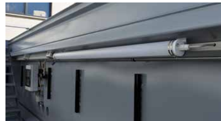
LED tube luminaire, 1630 mm long, 3800 lm
