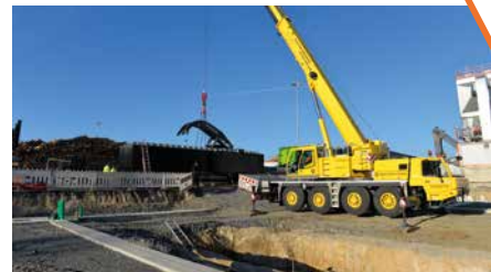
The TRUCKBAY is lifted in one piece with a crane to its destination.
