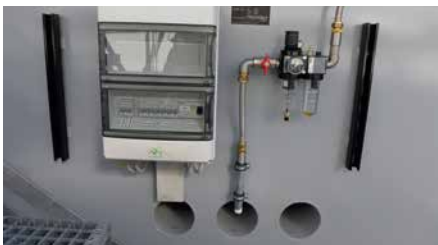
All the necessary supply lines are routed and connected.
