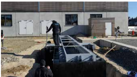
The TRUCKBAY is levelled before casting.
